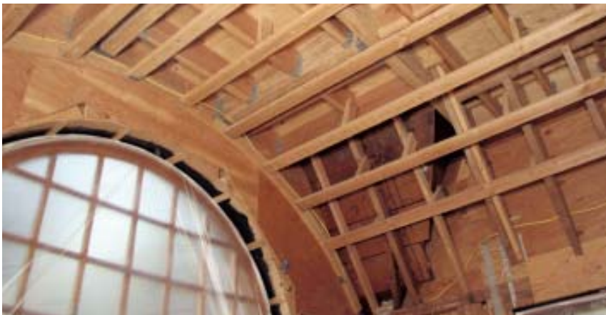
Figure 4. This barrel ceiling (above) would be difficult to insulate and seal with traditional materials. It's an ideal candidate for spray foam, which conforms to its irregular surfaces (left).
