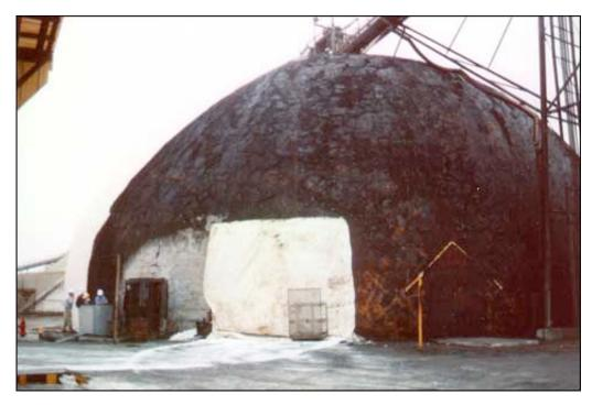
Outline of the wood building against the Monolithic dome. When the char from the  $2 \times 4$ 's was cleaned off, it left the outline of the wood structure. You can see where the foam was burned totally off the concrete, exposing rebar hangers and bases. This is the area of the 300 gallons of transformer oil that was totally consumed.
